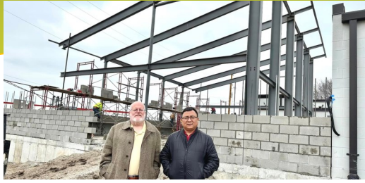
Multipurpose Center construction in progress
